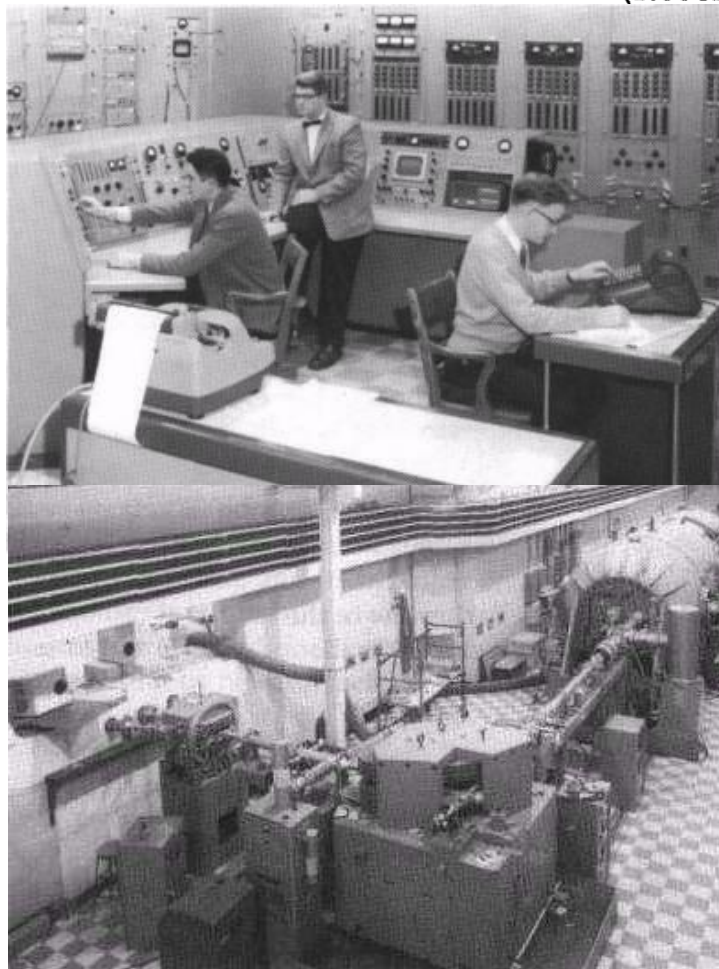
The world's first tandem accelerator installed at Chalk River in 1959.
